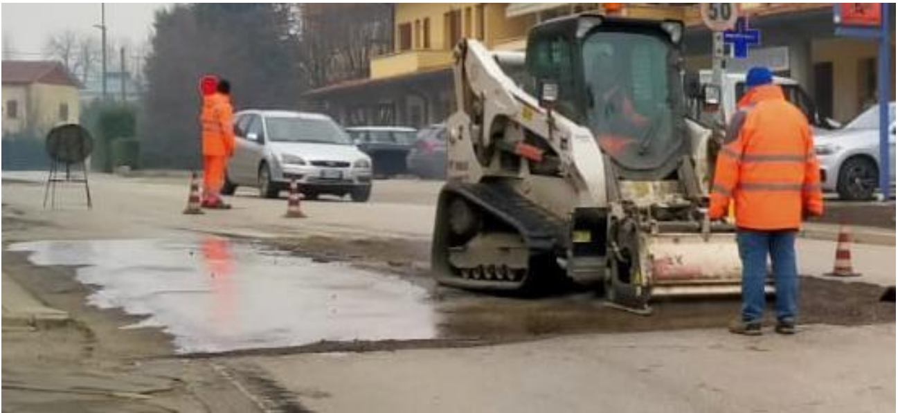
POLYGEN NANO ADDED DIRECTLY ON THE MILLED ASPHALT TO BE REGENERATED
