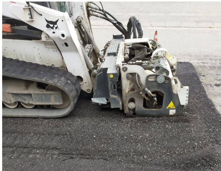
MIXING POLYGEN NANO WITH MILLED ASPHALT
