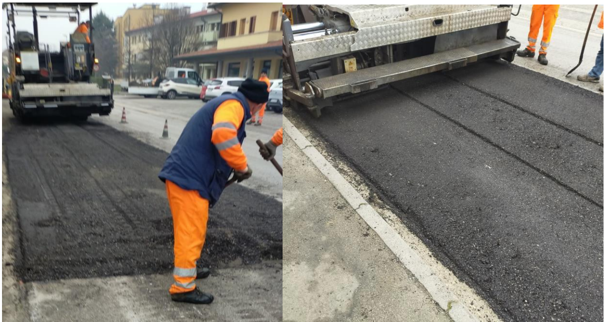
OPERATION - MILLED ASPHALT ADDED WITH POLYGEN NANO
