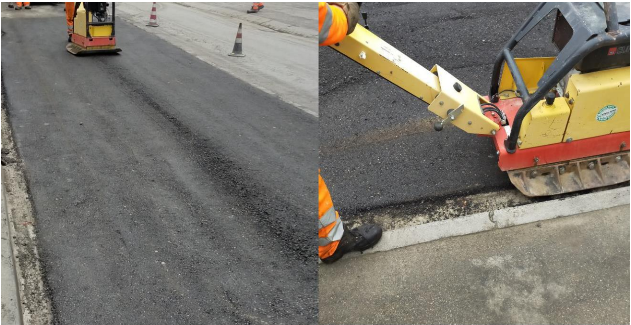
COMPACTION OF THE FINAL ASPHALT LAYER
